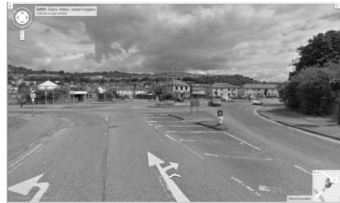
Unappealing, traffic dominated area with no sense of identity - no sense of entering a village/town and no awareness of the high quality urban area further along the road
